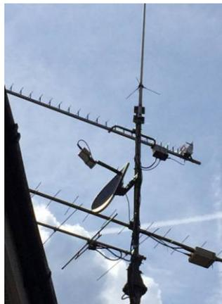
A long yagi or beam is needed to work any distance and in order to achieve reasonable results on any band it is essential to use a mast head pre-amplifier. The latest generation of MMICs mean that a sub 1dB noise figure and very good cross modulation performance can be achieved from very simple designs which are easy to build and
